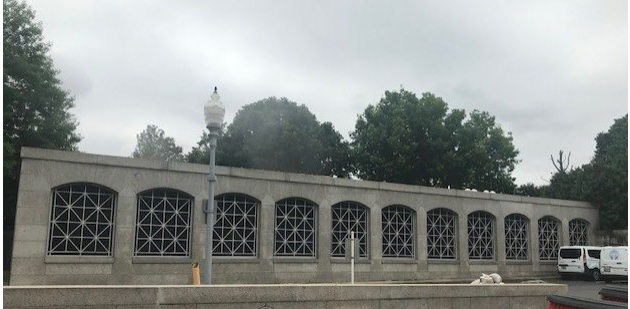
Existing Custom NMNH Cooling Tower
