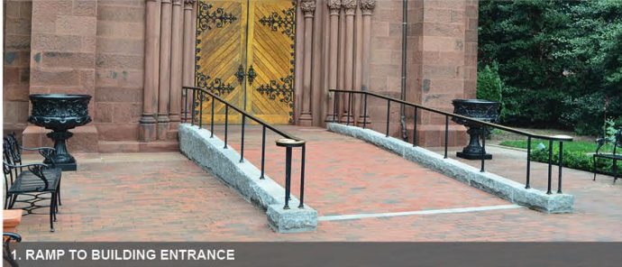
1. RAMP TO BUILDING ENTRANCE
