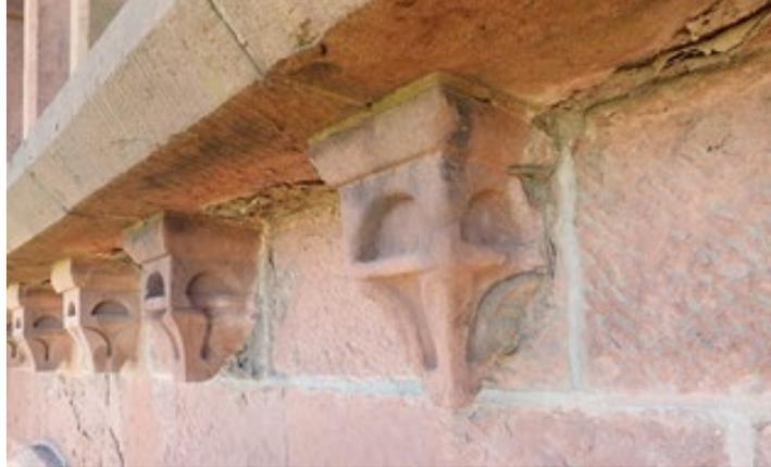
Masonry Damage Below Horizontal Projections
