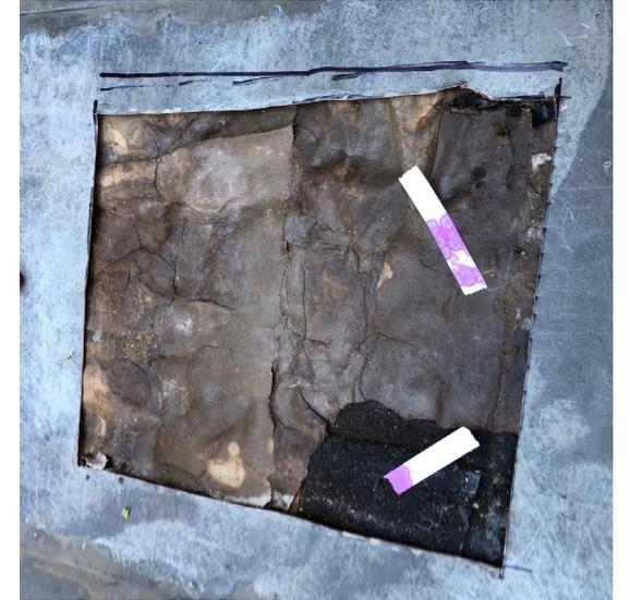
Water Below Copper Roofing, Typical
