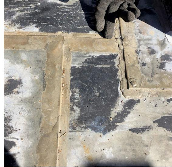
Typical Thin Solder at Seams in Copper Seams
