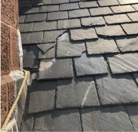
Typical Broken, Missing, or Loose Slate Shingles
