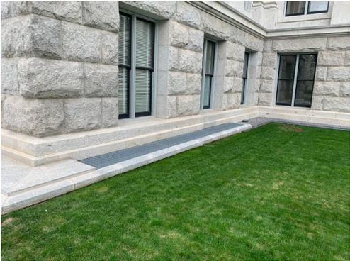
Integrated Seismic Joint Cover Examples
