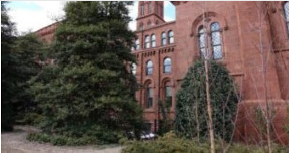
Existing southeast façade.
