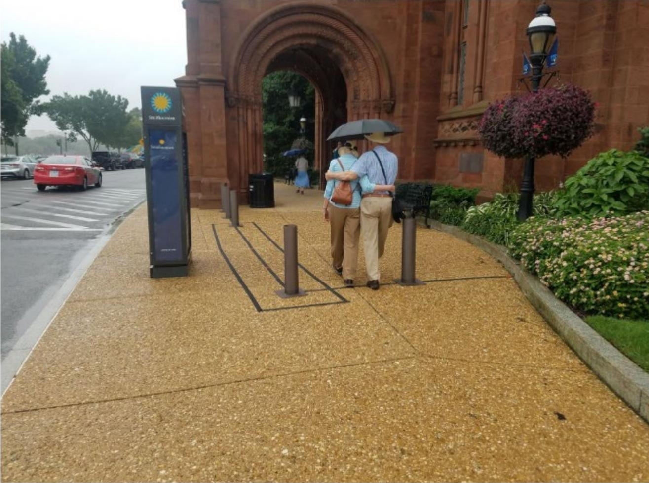
Conceptual bollard configuration at west side of porte-cochere with hardened bench massing taped-out on pavement
