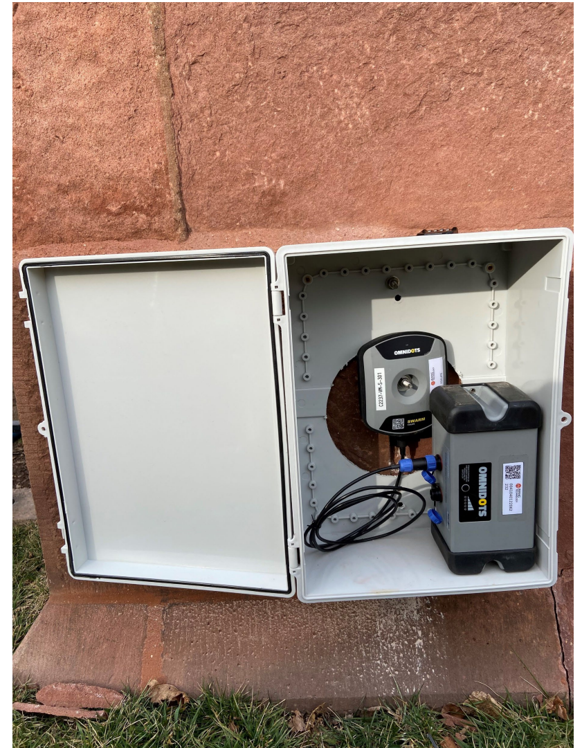
Vibration Monitor on the South Elevation, January 2023.
