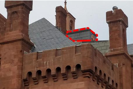
Southeast roof. Existing elevator penthouse to be removed (shown in dashed red lines).
