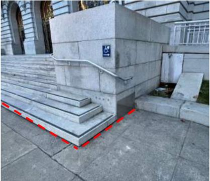
*Example of Seismic Joint Below Bottom Tread of Stair*
