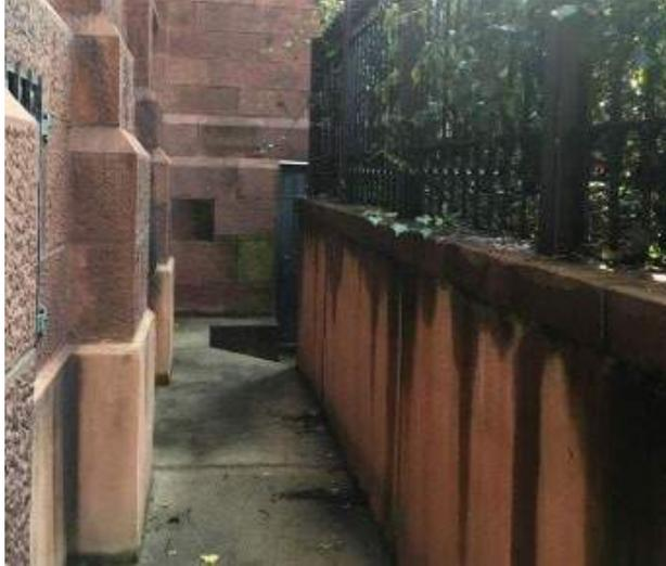
View of SW areaway – new walls were constructed of new tinted concrete while exposed foundations were parged
