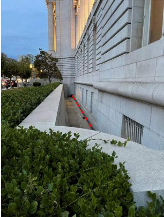
*Example of Areaway With Vertical Seismic Joint at Wall*
