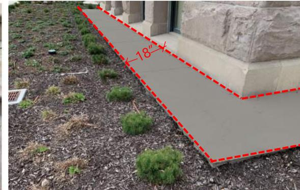
Integrated Seismic Joint Cover Example – Salt Lake City County Building
