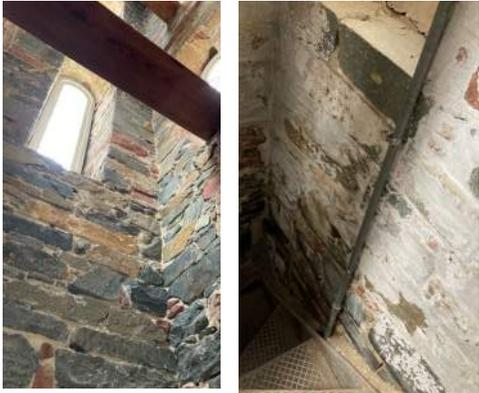
Examples in SIB showing the existing rubble stone and/or brick wall construction
