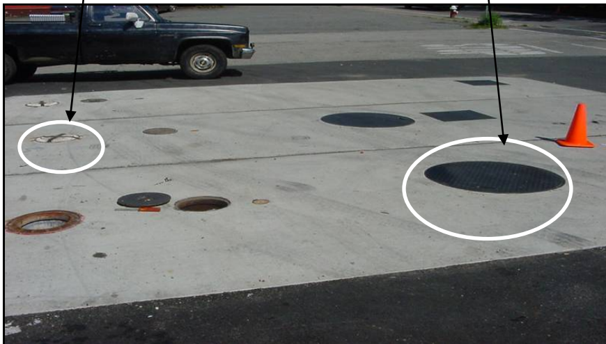
View of sump lids
